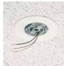
5 Pull cable. Install fixture per manufacturer's instructions.
