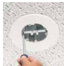
4 Add bracket to inside of box.
