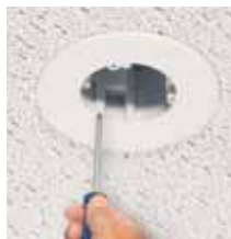
2 Install CAM-LIGHT box. Rotate to desired position. Tighten mounting wing screws.
