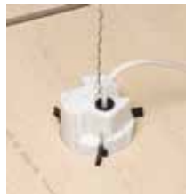
4 See steps 1-3 above. Install NM cable connector (supplied).
