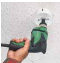
1 Cut hole in ceiling tile w/ 4" hole saw.
