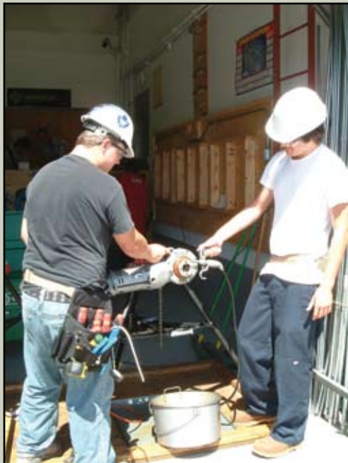
JAC Pre-Apprentices using power threader on rigid conduit
