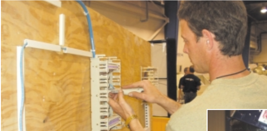
Punching down the Network Cabling Specialist project.
